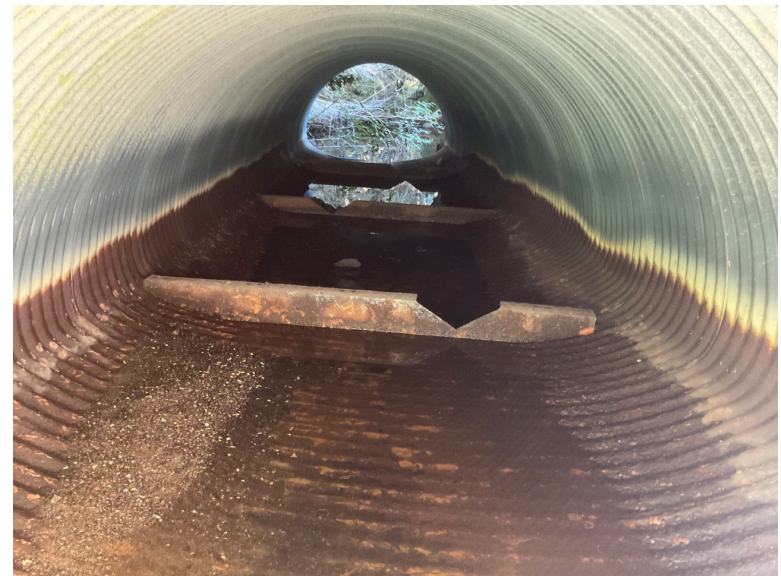
Looking Downstream Through CMP
